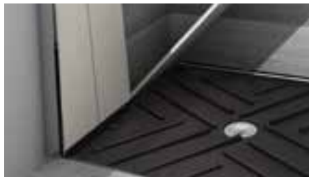
VERIFICATION OF THE INSTALLATION
