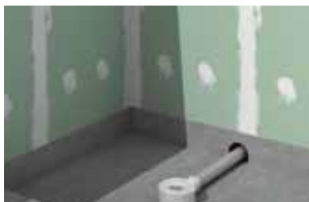
CONNECTION OF THE DRAIN
