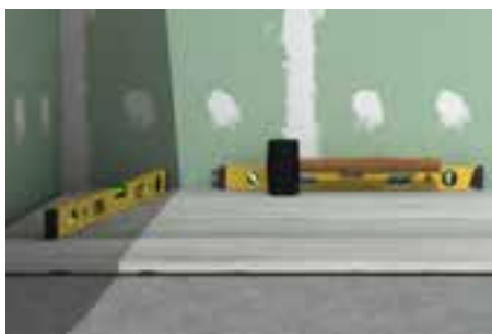
INSTALLATION OF THE SHOWER TRAY
