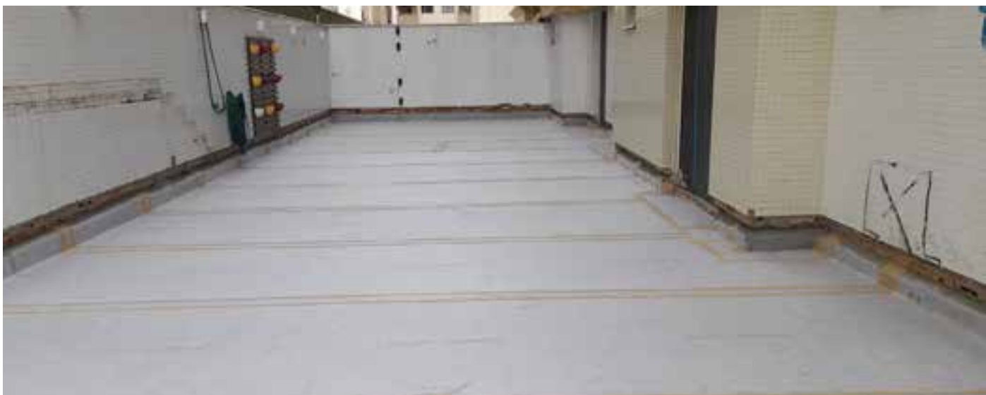
Waterproofing of 700 m 2 with ECODRY120 on all its outdoor walkable terraces. Condo in Itapema. Brazil.
