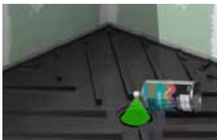
POSITION OF THE DRAIN
