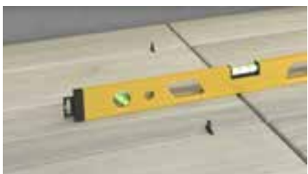
INSTALLATION OF THE BATHROOM FLOOR
