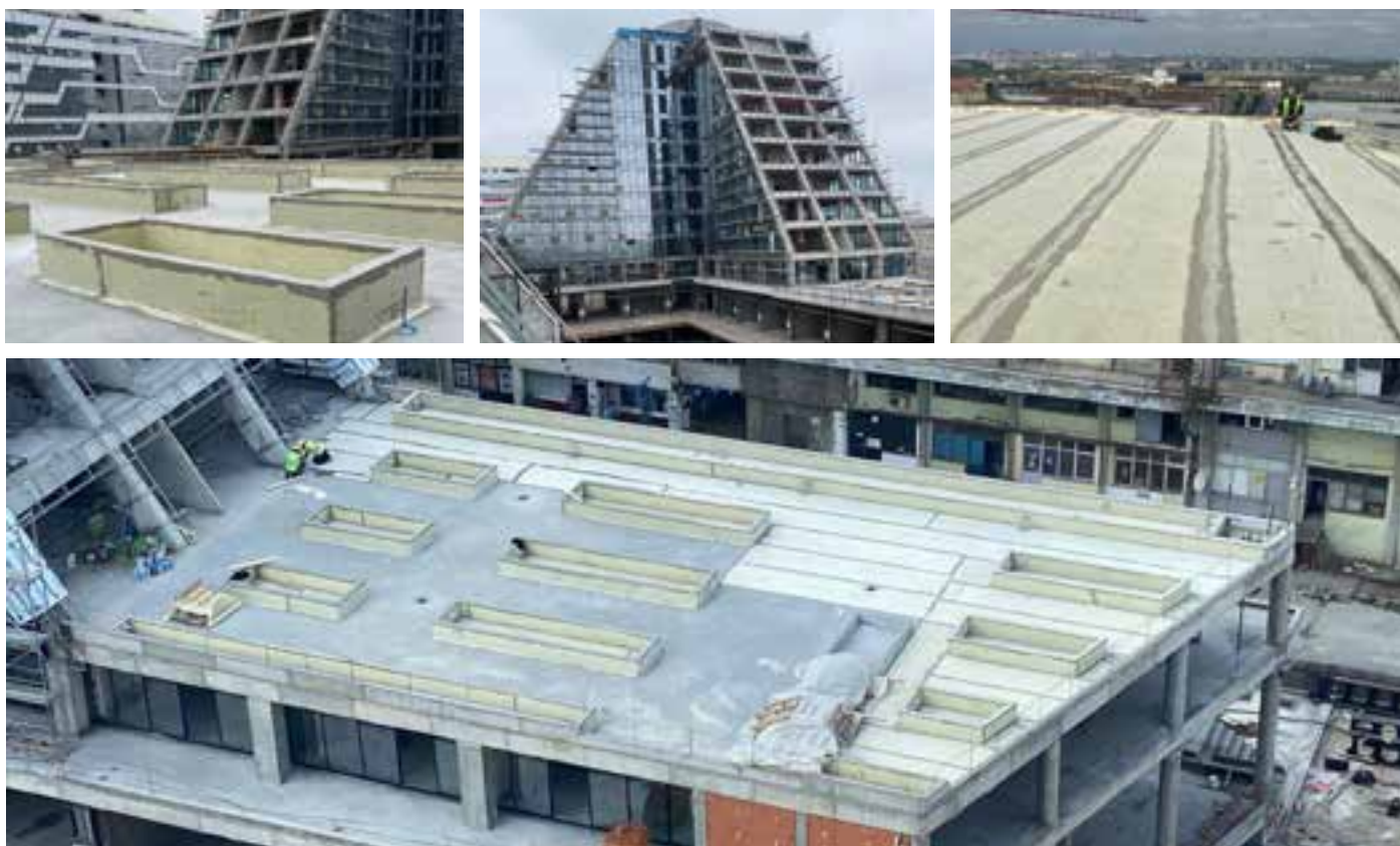
Waterproofing of 20.000 m 2 of DRY40 and DRY120 in all its outdoor walkable terraces. ISTMALL ISTANBUL. Building for offices, university and shopping center. Istanbul. Turkey.
