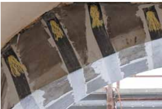
Detail of the U-wraps and ARMOGRIP connectors
