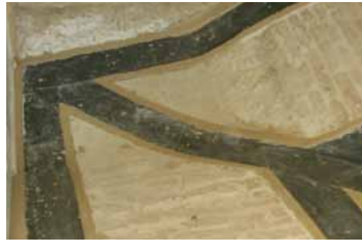
Particular of the points of connection between the vault and the perimeter wall
