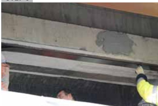
Application of ARMOSHIELD CFK plate along the length of the beam
