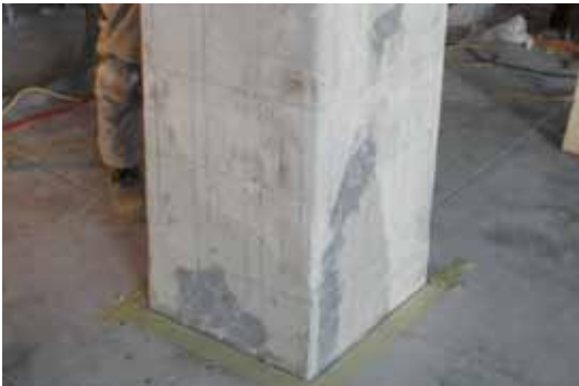
Volumetric rebuilding of the pillar with reinforced mortar of FLUECO line
