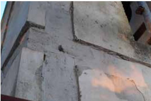
Preparation of the grooves for the housing of fabrics (*)
