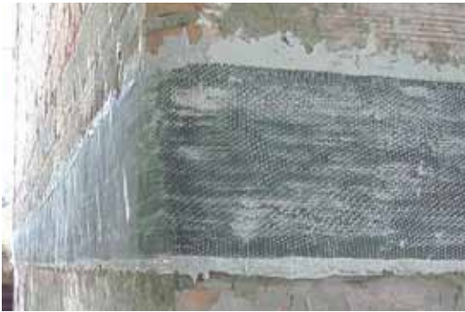
Wrapping with unidirectional fabric: detail of the rounded corner
