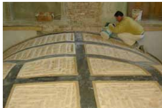
Overview of the reinforcement applied to the extrados and nearing completion
