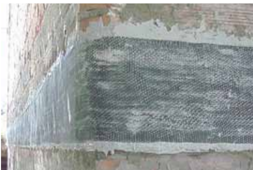
Wrapping with ARMOSHIELD C unidirectional carbon fibre fabrics
