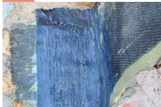
Portion of carbon fibre fabric applied on the thread to protect the connector
