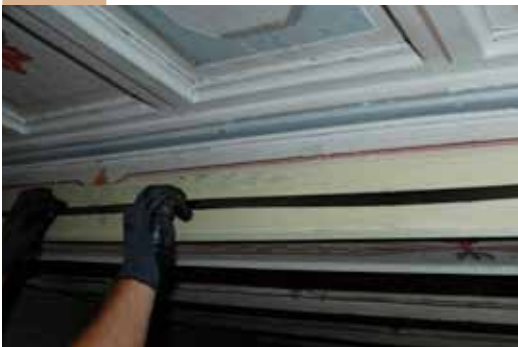
Insertion of ARMOSHIELD CFK plate
