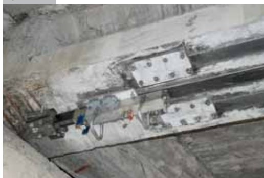
Plate pre-tensioning with hydraulic jack
