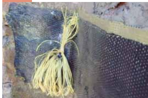
Insertion of the aramid connector ARMOGRIP BC inside the hole filled with ARMOFIX MTX resin
