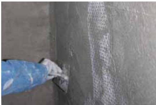
The mesh is applied between two coats of ARMOTECH MONO mortar.
