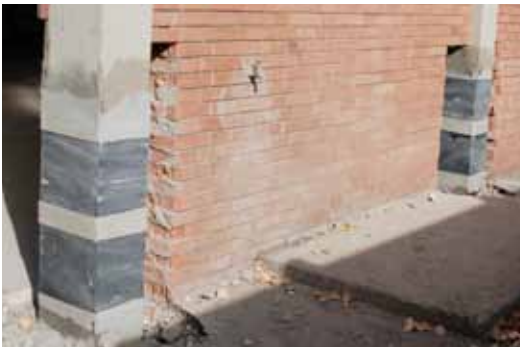
Overview - Reinforced concrete pillars with ARMOSHIELD C-SHEET carbon fibre fabric
