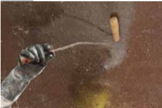
Lay the epoxy primer ARMOPRIMER 100 by brush to promote adhesion
