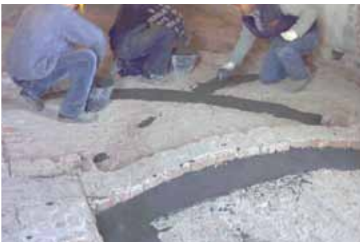
Application of the resin for bonding
