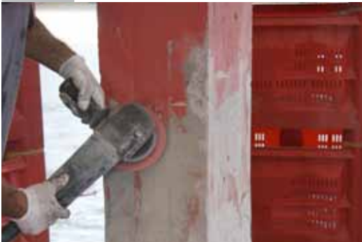
Removal of the existing coating and surface cleaning
