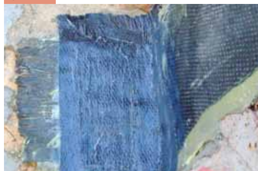
Portion of ARMOSHIELD C carbon fibre fabric applied on the thread to protect the connector
