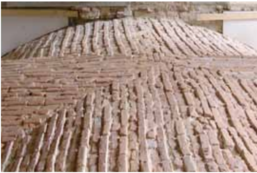
The groin vault before the intervention after cleaning
