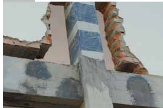
Wrapping of the pillar with ARMOSHIELD C carbon fibre fabrics
