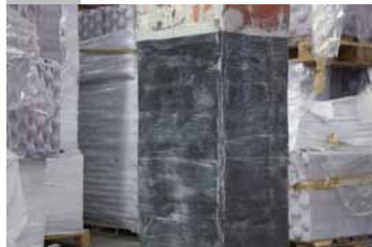
Complete wrapping around the entire perimeter of the pillar
