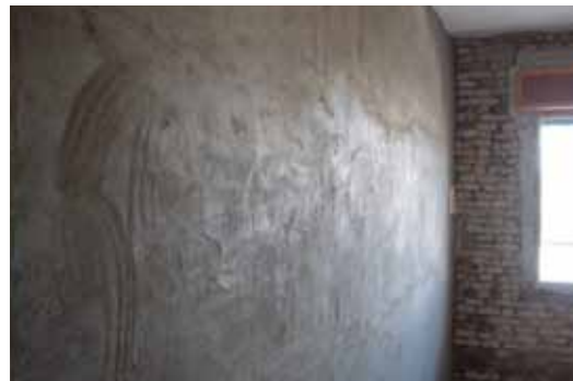
The anti-overturning intervention has been accomplished
