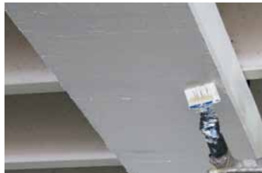
Protective finishing with plaster or with other cement or resin coatings
