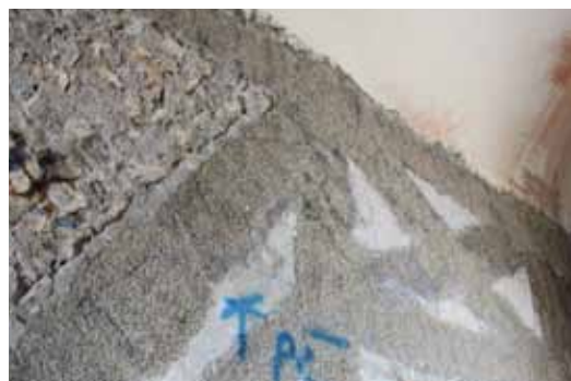
Quartz sand sprinkle promoting the subsequent plaster application
