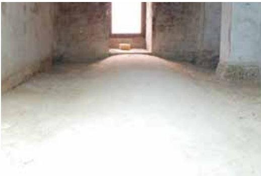
The barrel vault before the intervention: removal of the surface coating
