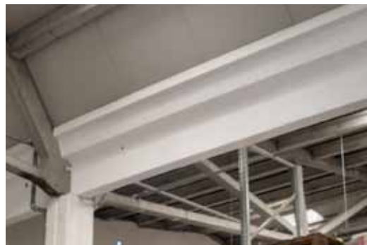
Application of protective coat
