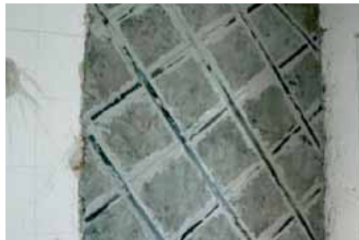
Braces made with ARMOSHIELD CFK carbon fibre plates
