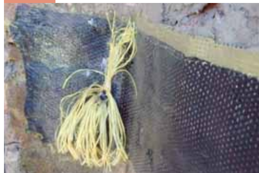
Insertion of ARMOGRIP BC aramid connector
