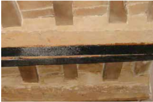
Application of ARMOSHIELD C SHEET carbon fibre fabrics to the intrados of the beam
