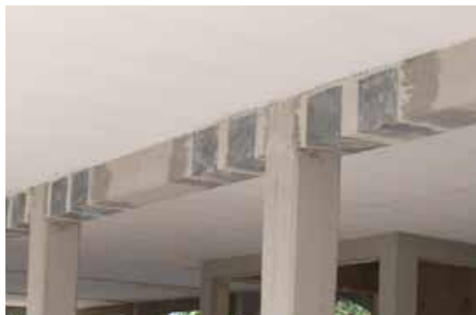
Overview - Fabrics are applied close to supports
