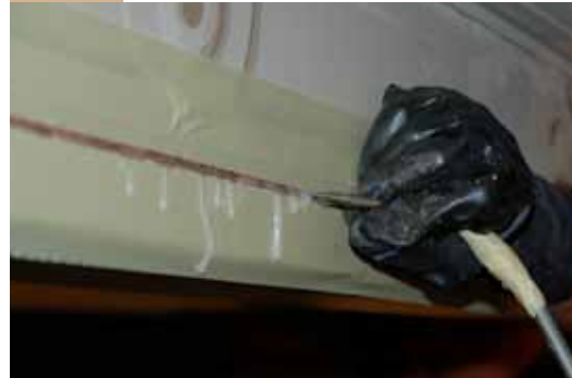
Injection of ARMOFIX MTX adhesive
