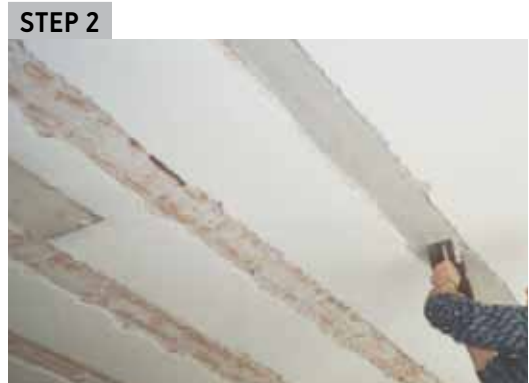
Application of ARMOFIX MTL epoxy resin, ideal for plate bonding
