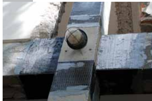
The confinement intervention has been accomplished
