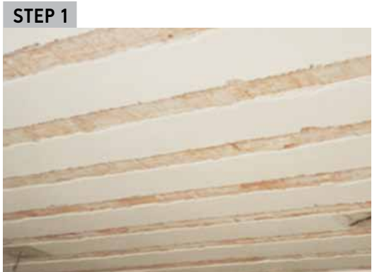
Demolition of the joist bottom and surface cleaning
