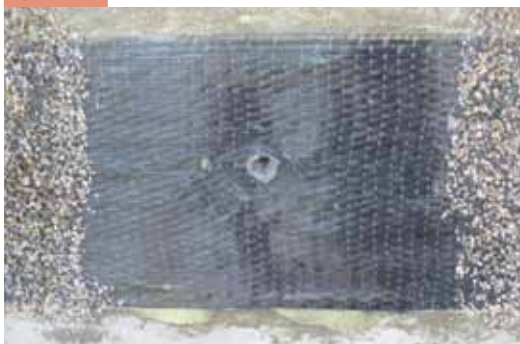
The fibres of carbon fabric must be carefully spread at the holes
