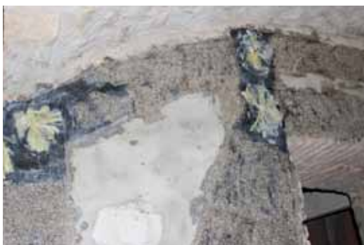
Interconnections with ARMOGRIP double-thread aramid connector
