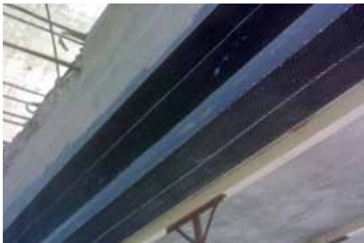
Application of ARMOSHIELD-C carbon fibre fabrics to the intrados of the beam
