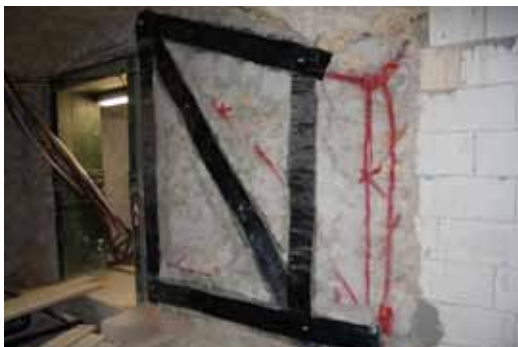
Fabric application on the mortar grooves
