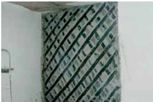
Braces made with ARMOSHIELD C unidirectional carbon fibre fabrics
