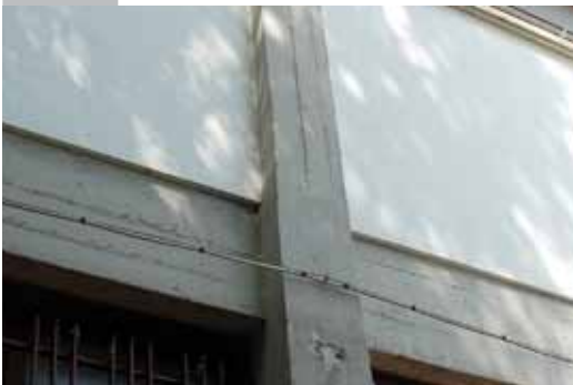
Beam-pillar junction before the intervention
