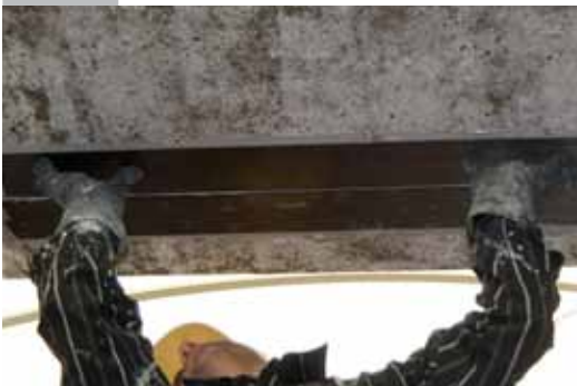
Lay ARMOSHIELD CFK plates over the fresh resin coat
