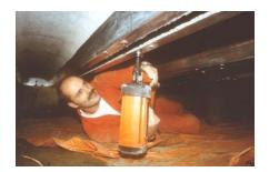
3. By using screw anchor like fasteners (so called tapcons), which can be applied directly into concrete. Be aware of pre-drilling the holes with the appropriate drill bit diameter.
