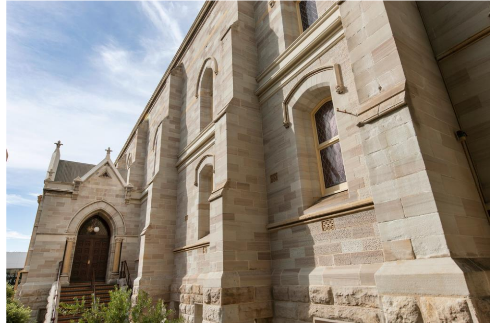
Restoration works on Elder Hall
