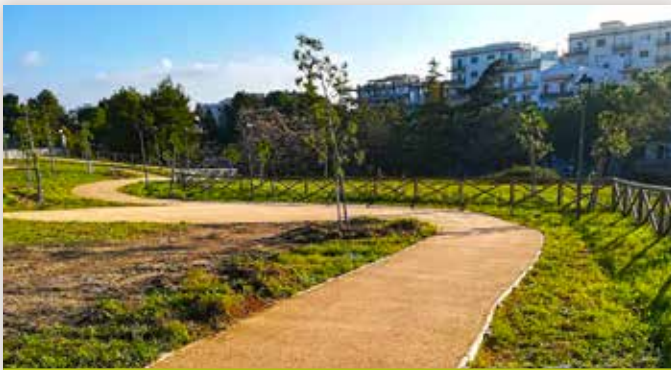
CRISPIANO (TA) - Redevelopment of the Gravine Vallone Area Cycle and pedestrian paving (2018)
