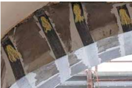
Detail of the U-wraps and ARMOGRIP connectors
