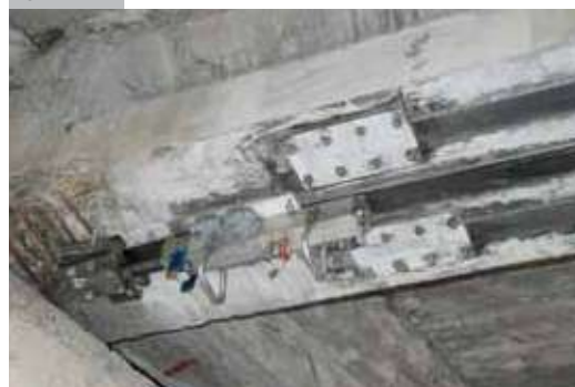
Plate pre-tensioning with hydraulic jack
