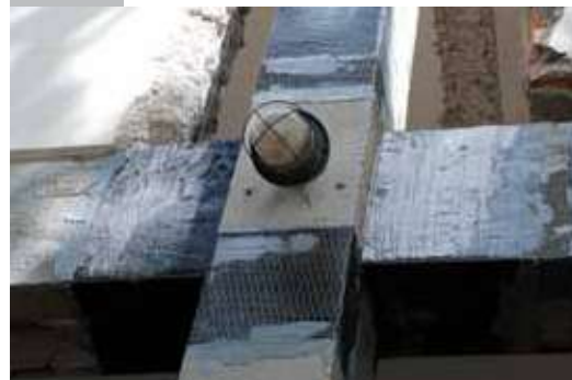
The confinement intervention has been accomplished
