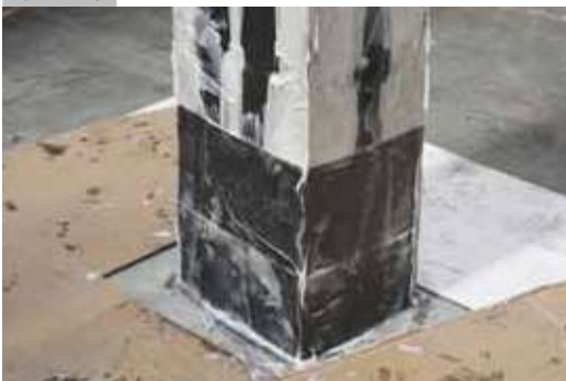
Laying of ARMOSHIELD C-SHEET unidirectional fabrics on ARMOFIX MTX resin and impregnation
