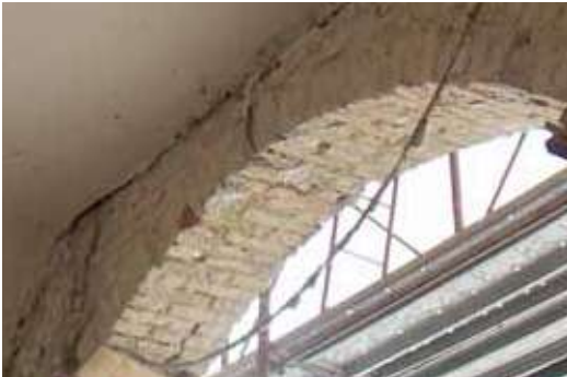
The arch before the intervention: complete removal of plaster or existing coatings
