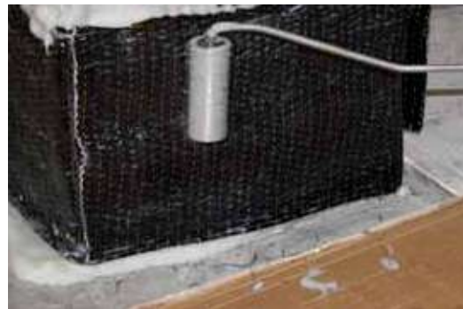
Laying of ARMOSHIELD C-SHEET fabric and impregnation with ARMOFIX MTX epoxy resin
