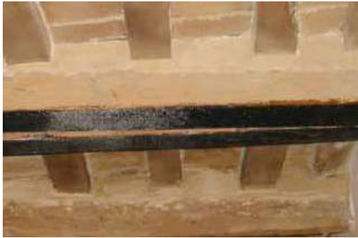
Application of ARMOSHIELD C SHEET carbon fibre fabrics to the intrados of the beam
