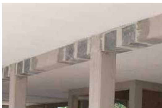
Overview - Fabrics are applied close to supports
