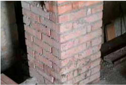
Compressed masonry pillar before intervention
