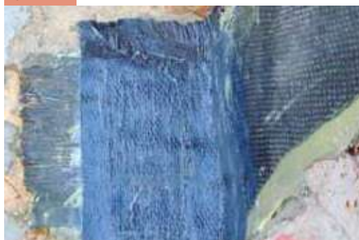
Portion of ARMOSHIELD C carbon fibre fabric applied on the thread to protect the connector
