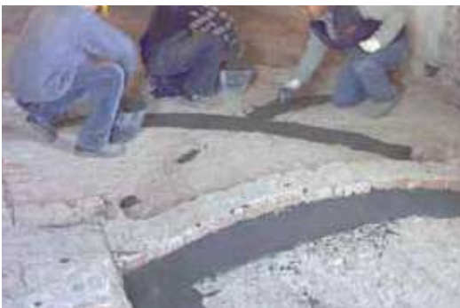
Application of the resin for bonding
