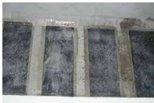
Application of ARMOSHIELD C-SHEET fabrics over the fresh coat of ARMOFIX MTX resin
