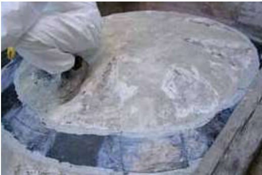
Application of ARMOSHIELD fabrics on the mortar grooves
