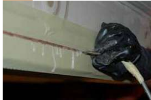
Injection of ARMOFIX MTX adhesive
