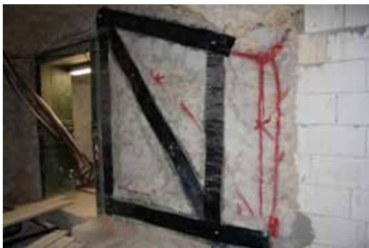
Fabric application on the mortar grooves
