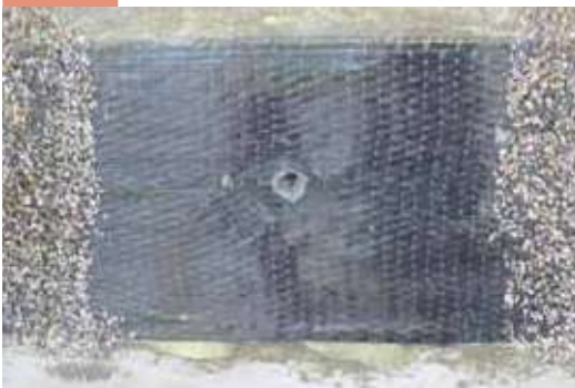
The fibres must be carefully spread at the holes
