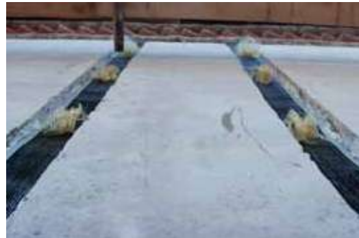
Laying of ARMOSHIELD C carbon fibre fabrics on the mortar housing grooves and insertion of ARMOGRIP connectors
