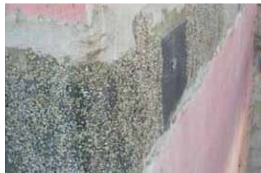
Detail of the final quartz sand sprinkle promoting the subsequent plaster application
