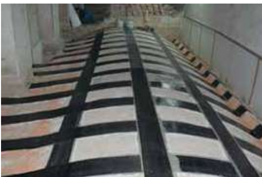
Application on the extrados
