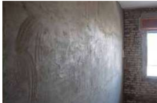
The anti-overturning intervention has been accomplished
