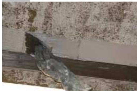
Apply the epoxy adhesive ARMOFIX MTL, ideal for plate application.
