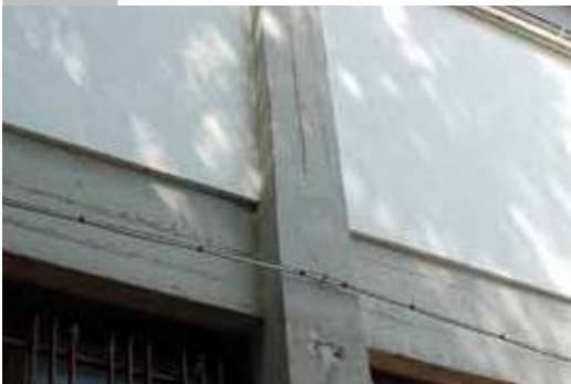
Beam-pillar junction before the intervention
