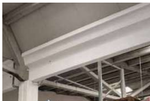
Application of protective coat
