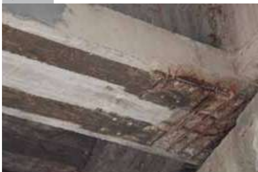
Drilling of the holes for plate anchoring and application of ARMOPRIMER 100 primer
