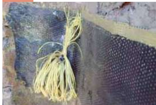
Insertion of ARMOGRIP BC aramid connector
