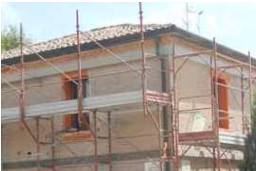
Overview of the intervention: wrapping performed at the top and at the floor slab
