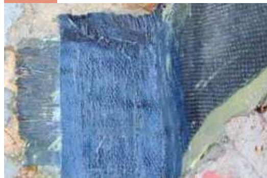
Portion of carbon fibre fabric applied on the thread to protect the connector
