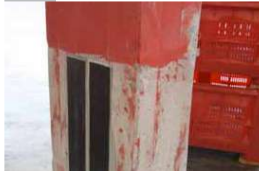
Application of ARMOFIX MTL epoxy adhesive for bonding and ARMOSHIELD CFK plates
