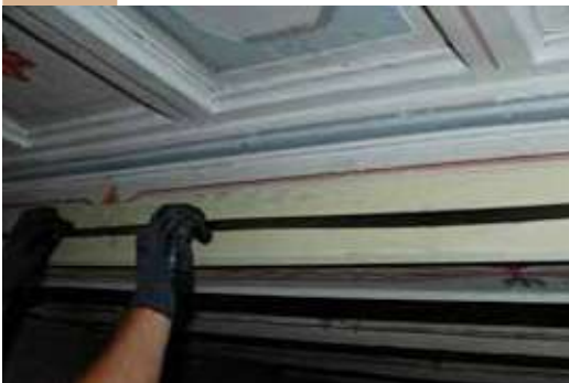
Insertion of ARMOSHIELD CFK plate
