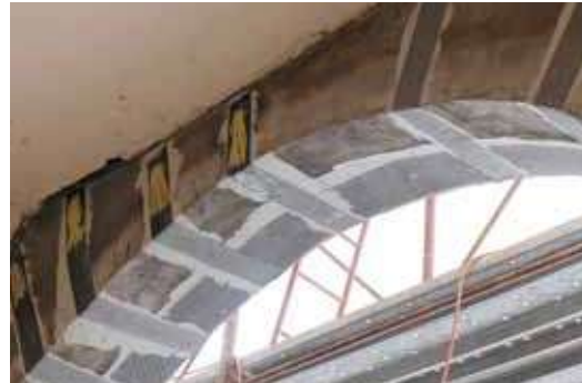
Application of ARMOSHIELD C-SHEET fabrics to the intrados and wrapping secured with ARMOGRIP connectors.
