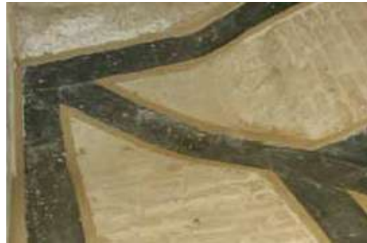
Particular of the points of connection between the vault and the perimeter wall
