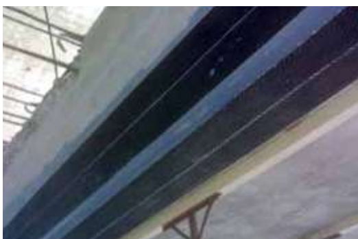
Application of ARMOSHIELD-C carbon fibre fabrics to the intrados of the beam
