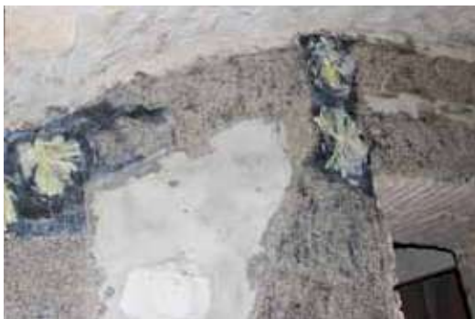
Interconnections with ARMOGRIP double-thread aramid connector
