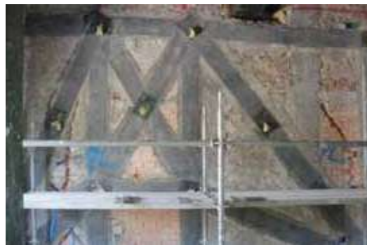
Wall reinforced on both sides with ARMOSHIELD C carbon fibre fabric placed according to the project model
