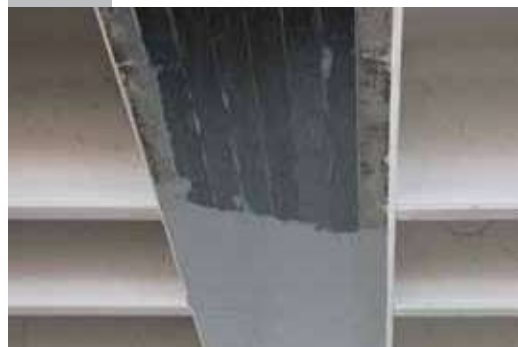
Apply ARMOFIX MTX adhesive over the plates until they are completely covered.
