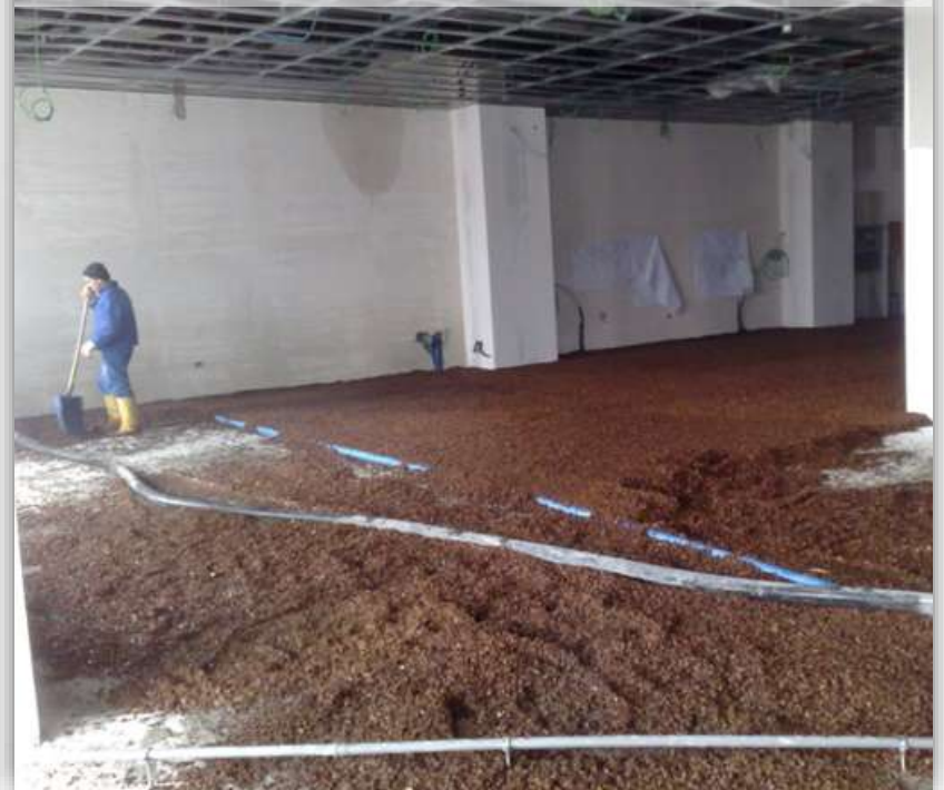
Leveling and smoothing the cork-made screed
