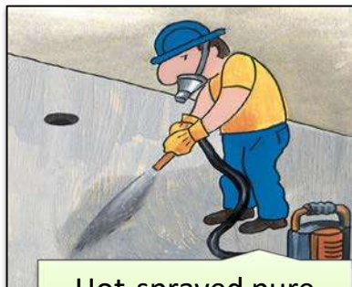
Hot-sprayed pure polyurea
