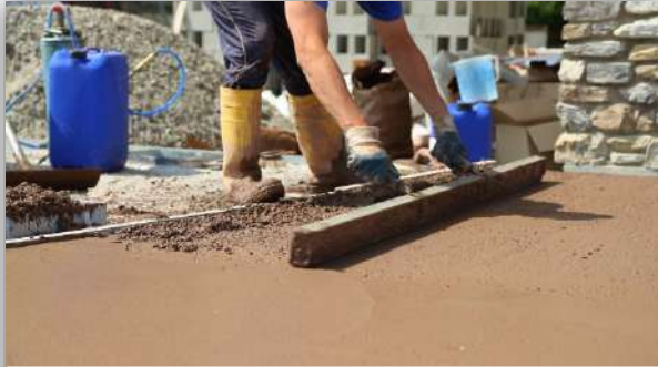
Normal flooring construction
