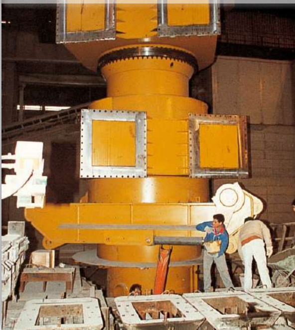
Anchoring of a piece of machinery in a steel-production plant
