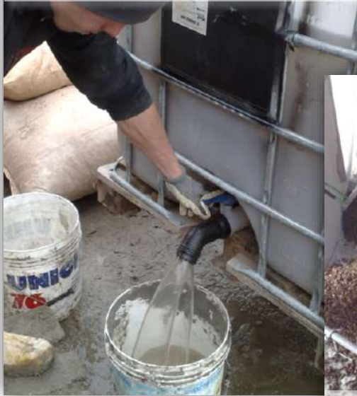
Dosing SANAGLAS (about 80-100 kg for every m 3 of cork)
