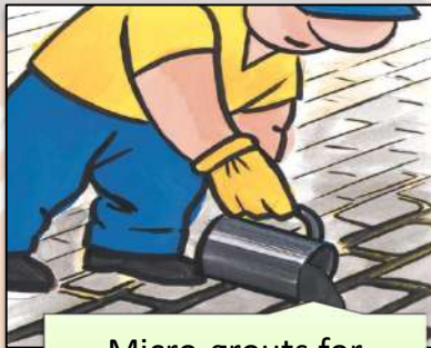
Micro-grouts for cobblestone roads
