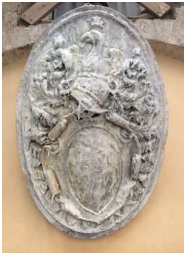
CLEANING WITH POLITECT AMMONIO CARBONATO 4%
