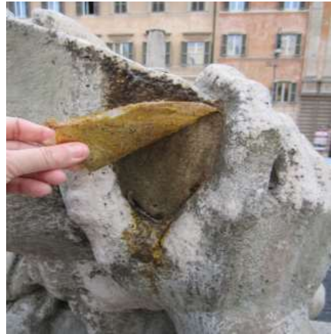
REMOVAL ( NOTICE THE SPORES RETAINED IN THE POLYMERIC FILM) BEFORE RINSE
