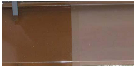
Part of an old and bleached Aluminium façade, following a clear coating.
