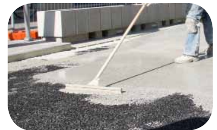
Laying DRACOBIT by a rubberized spatula
