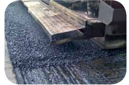
Lay an asphalt drainage mat
