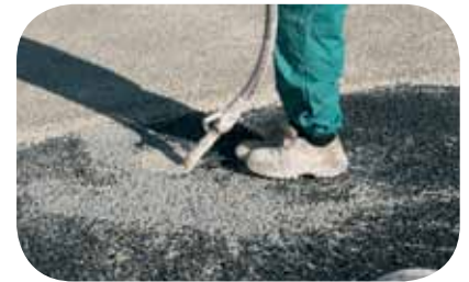
Saturation of the drainage mat
