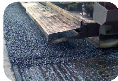
Application of the drainage layer
