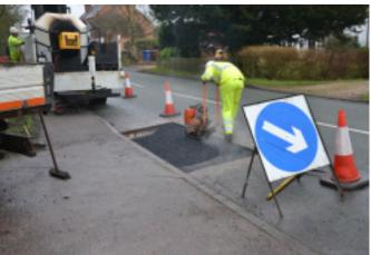
The hot Armaphalt material used as normal to complete the re-instatement.
