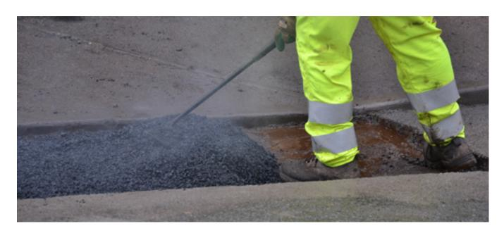
The hot Armaphalt material is ejected from the mixer ready to lay.
